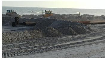
Our Storm Damage Reduction Project continues in full swing as Weeks Marine worked throughout the holiday to keep the dredging and sand placement moving forward. The dredge *Borinquen* completed its work in Topsail Creek and the "Cut Through" Channel near the inlet for safer and quicker access. Sand placement on the beach started
